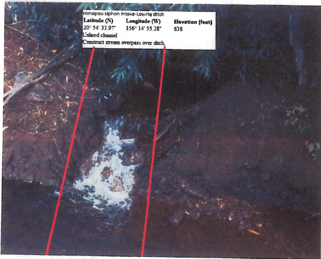
Photo 3 (above): Honopou siphon at Lowrie Ditch (L-16)
