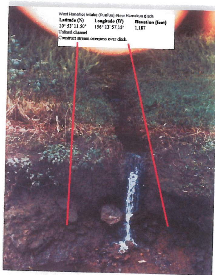
Photo 9 (above): Puolua (Huelo) at New Hamakua Ditch (NH-17a)
