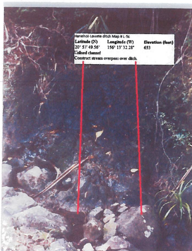
Photo 8 (below): Hanehoi small intake at Lowrie Ditch (L-5c)
