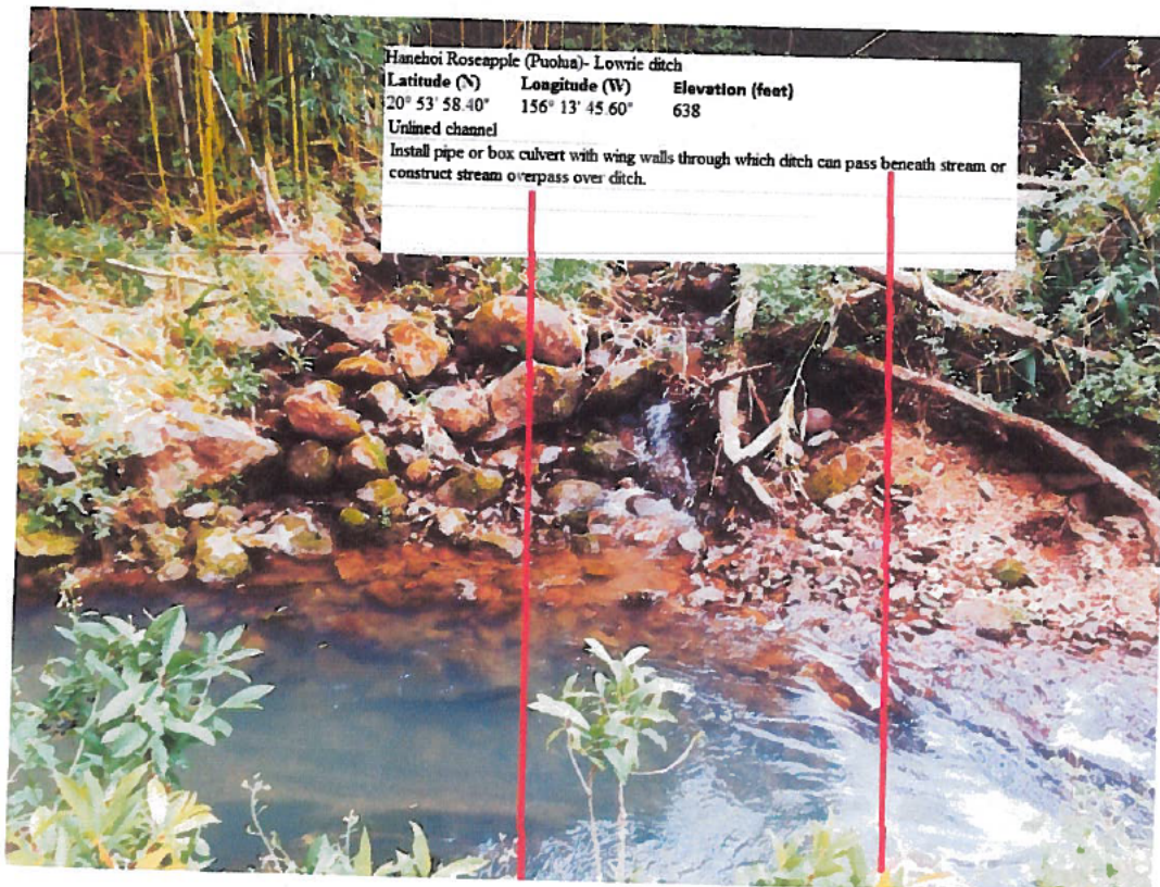
Photo 10 (below): Puolua (Huelo) at Lowrie Ditch (Hanehoi Roseapple) (L-7a)
